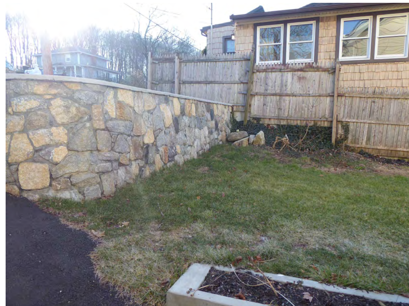
1 STONE RETAINING WALL WITH REPAIRS SCALE: 1/4" = 1'-0"
